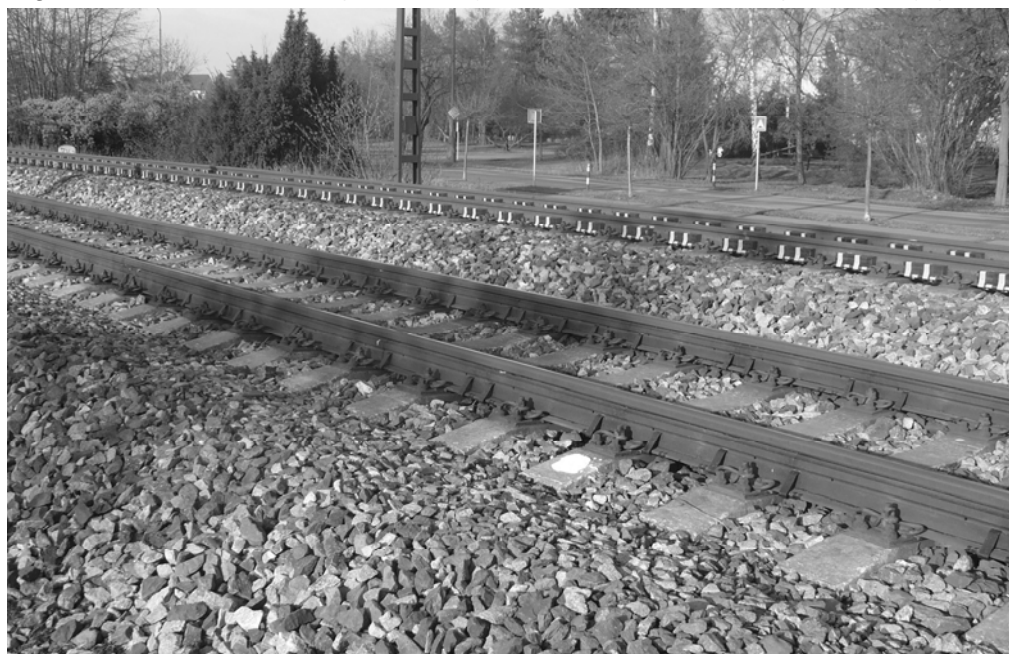
Fig. 2: Mounted Vossloh (Rail No. 1) and Corus absorbers (Rail No. 2) (December 2009)
